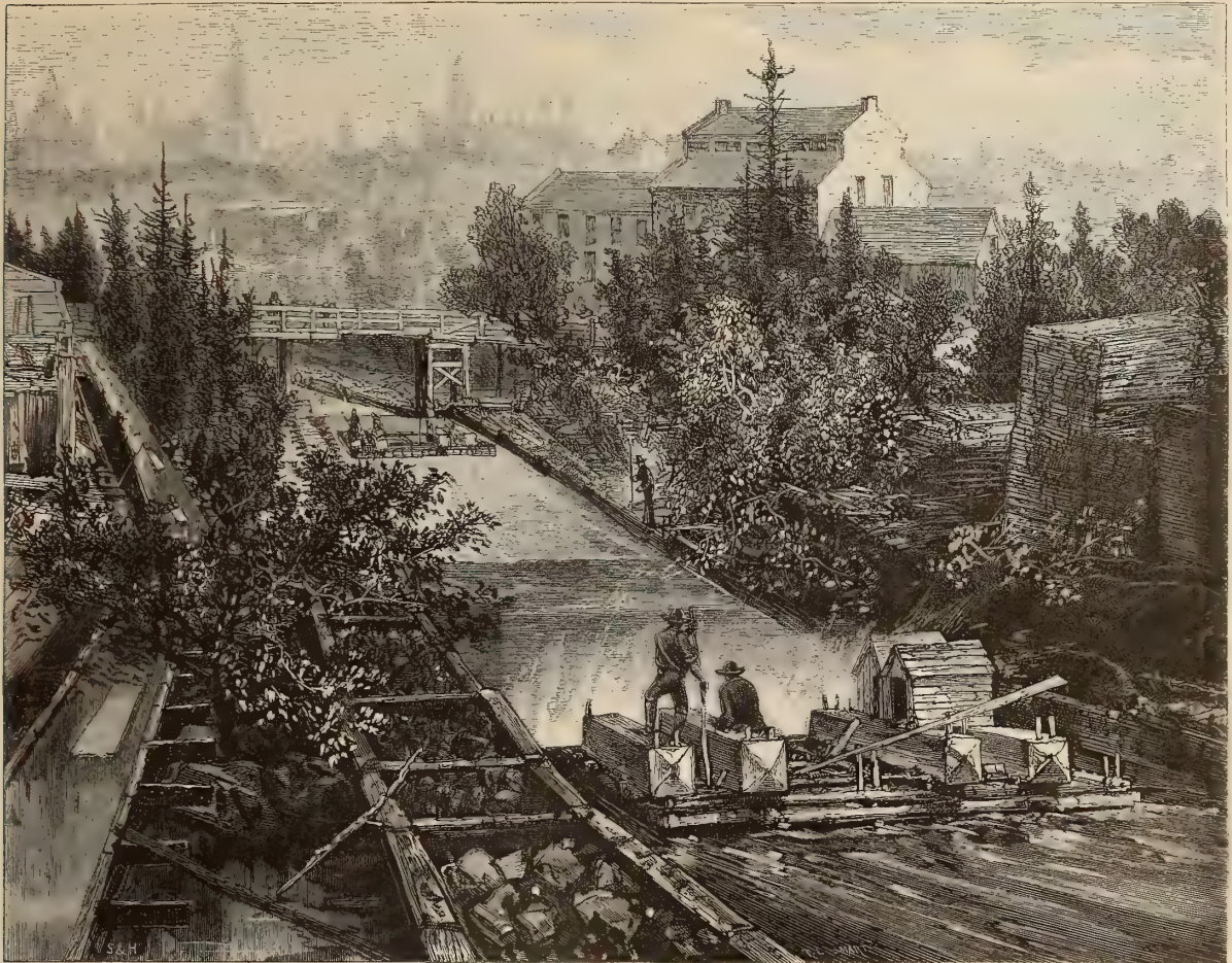
CRIB OF TIMBER RUNNING THE SLIDE.
